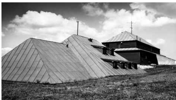
Extension to the Rýchorská bouda Chalet for the needs of the Centre for Ecological Education; still known at that time as the Educational Centre for State Nature Protection, opened in 1986 (photo Jiří Bruník)
