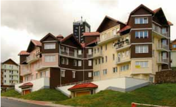
Apartments have filled most of the open spaces in the centre of Pec pod Sněžkou (photo Kamila Antošová)
