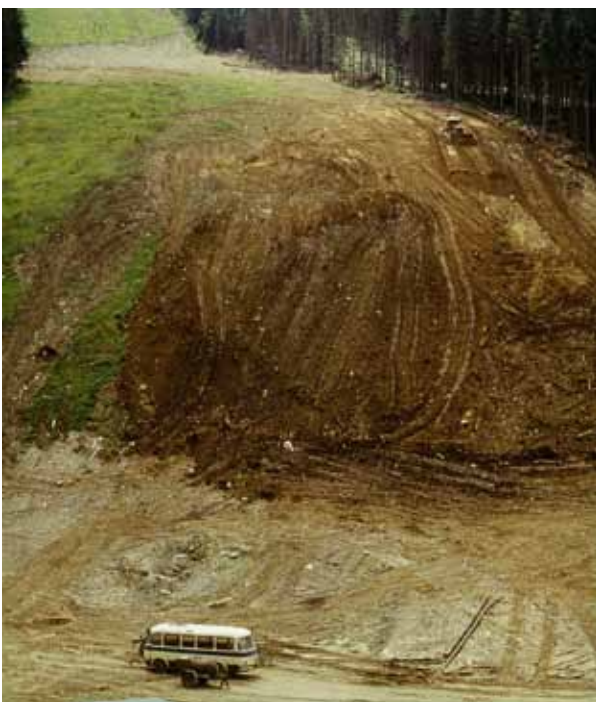
Insufficiently stabilised slope of the 'Great Drum' on the black ski slope at Svatý Petr during modifications in the 1970s (photo Jan Štursa)
