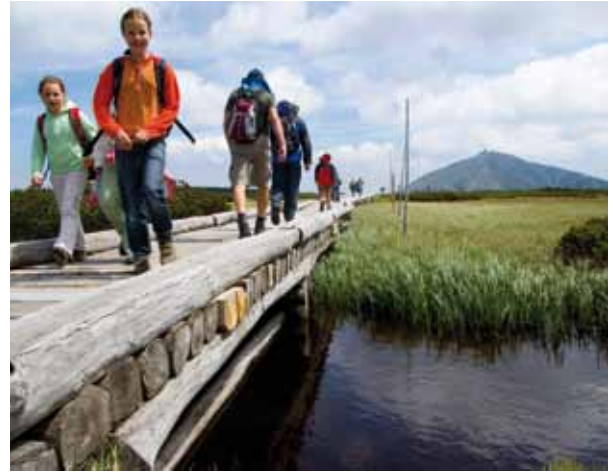
In place of the former limestone embankment, an oak-built wooden walkway runs across the revitalized Úpské rašeliniště Peatbog on piles (2009, 13 years after it was built, photo Kamila Antošová).
