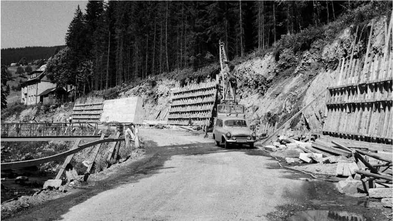
The series of reconstructions of main roads leading to the Krkonoše resorts and to the border crossings was begun in 1969. By 1979 the Horní Maršov—Pec pod Sněžkou (depicted here), Vrchlabí—Špindlerův Mlýn, Temný Důl—Pomezní Boudy and Kořenov—Harrachov roads were gradually widened by Polish construction companies. Later the Harrachov bypass was built – the more unnecessary the road, the wider it was built! (photo Miroslav Hladík)
