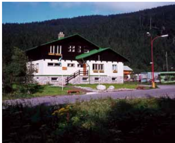
The Terrain Information Centre in Špindlerův Mlýn was opened in 1977 (photo Jiří Bruník)
