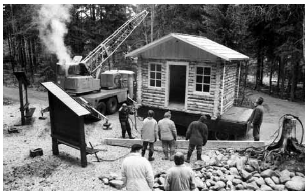
Installing the Terrain Service cabin at Dívčí lávky in October, 1994. In summer the cabin was to serve as an information point, in winter as a shelter for cross country skiers on the Keep Fit! Trail. Around the cabin are panels with educational texts, on the right the preserved roots around a spruce stump (photo Karel Hník)
