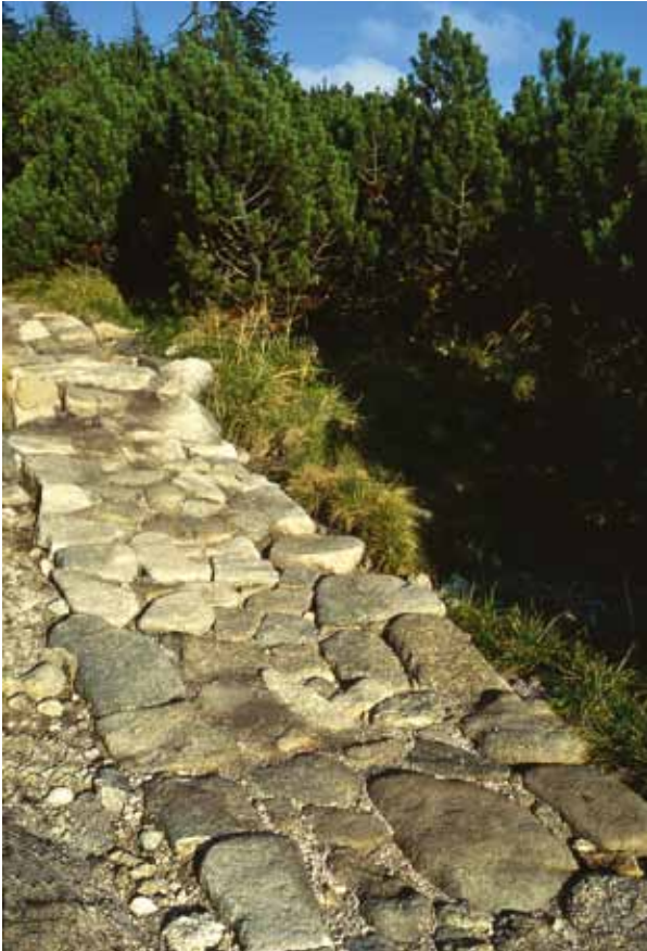
The stone pavement from the Labská bouda Chalet to the rim of the Sněžné jámy Cirques is evidence of sensitive work by today's mountain trail builders, following on from the traditional methods used by their predecessors (photo Jan Štursa)
