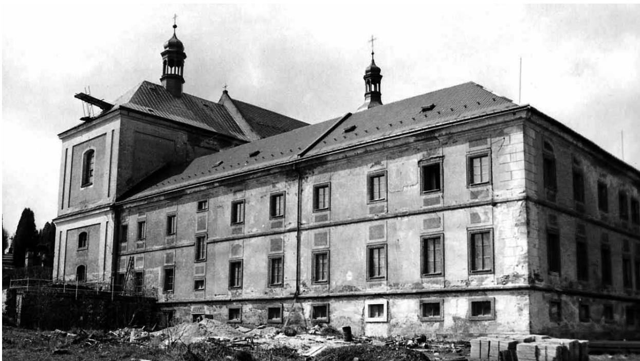
Since the 1950s the Museum of Krkonoše in Vrchlaví has occupied the Augustinian Monastery building. The KRNAP Administration took control of the museum in 1966 and carried out a demanding renovation project, which dragged on for 17 years (photo Jiří Bruník)
