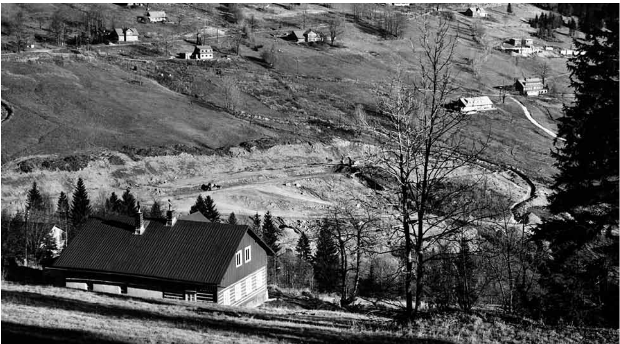
One of the most beautiful meadows at Labská (Zadní Krausovy Boudy Chalets) must give way to the Revolutionary Trade Unions' Pochodeň (Flaming Torch) Reconvalescence Home, completed in 1984 (later Arnika, today a private hotel). The deep gullies around the site are clearly visible - the water régime was irrevocably altered, the runoff rate was accelerated (photo Jiří Bruník)
