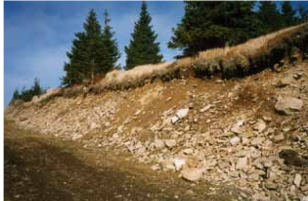
Detail from Mt. Medvědí: well- and badly-stabilised edges of the downhill ski runs. Slippage of rocks and collapses of the upper edge of the lateral slopes mean that their stabilisation takes many years to complete. This instability also complicates the maintenance of the ski slope and its safety in the early spring (photo Jan Štursa)
