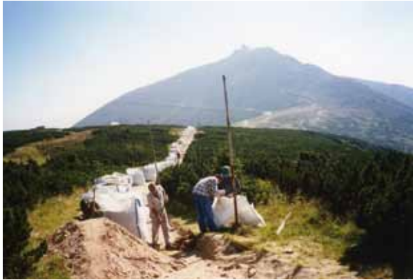
Sacks containing the remaining hundreds of tonnes of limestone from the trail from the Úpské rašeliniště Peatbog below Mt. Sněžka were removed by helicopter. This demanding reconstruction in 2001 was financed by the Ministry of the Environment from the Landscape Care Programme (photo Jan Štursa)
