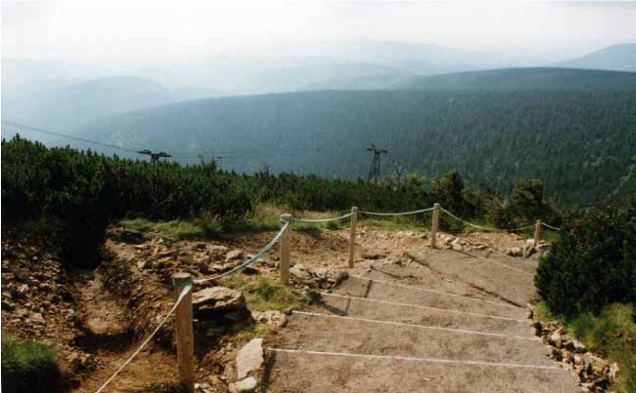
The system of transverse kerbstones and lateral drainage trenches prevents the erosion of construction materials from the pavement, by reducing the erosive strength of the surface water after heavy rain or from melting snow. However, regular maintenance work by the mountain trail builders is necessary to keep the pavement in good condition (photo Jan Štursa)
